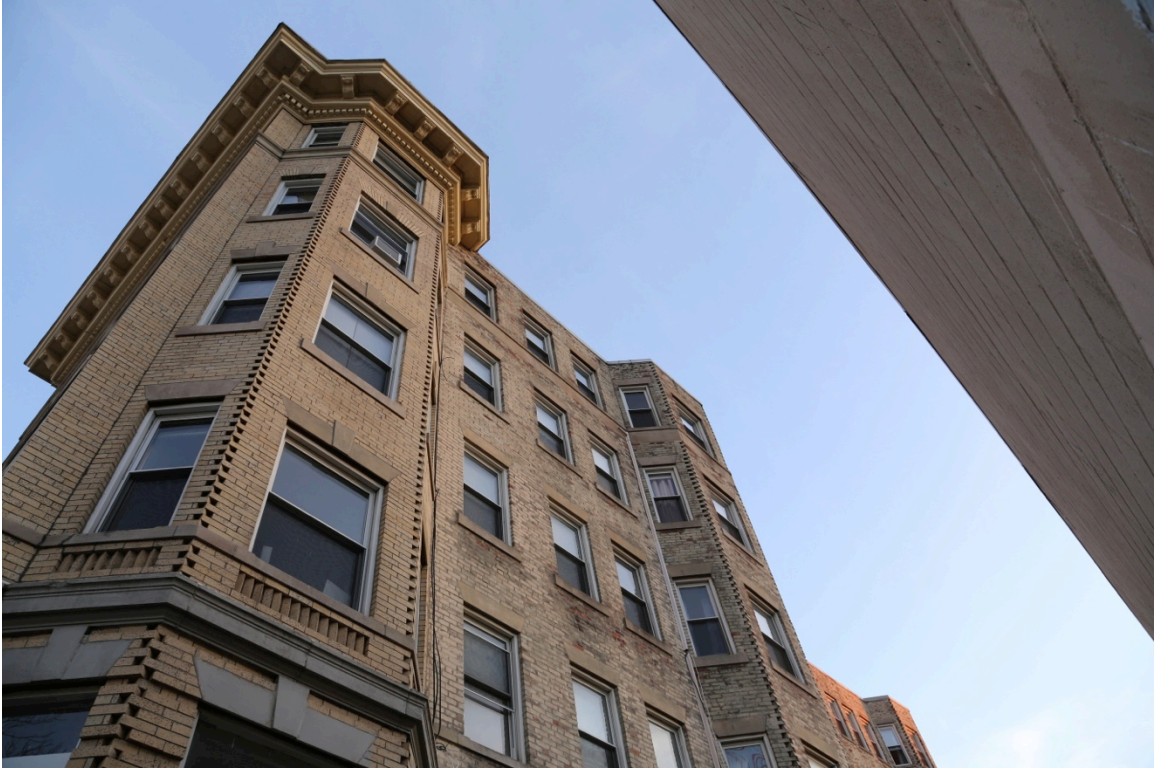
Figure 9. Original construction apartment building. Note how the crown molding roof decoration does not extend all the way around the building. Personal photograph.
