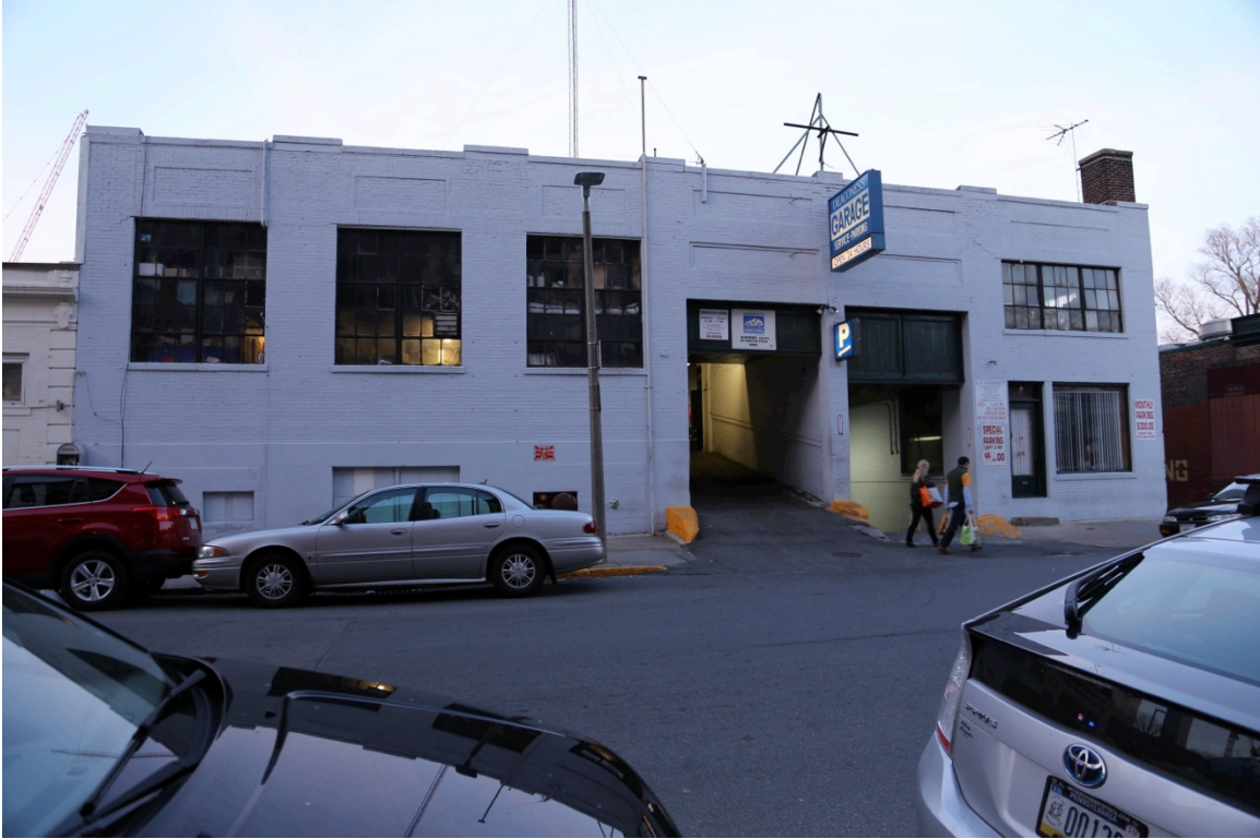
Figure 4. Taxicab service station and garage on the site. Likely virgin construction from the earliest development of the site. Personal photograph.
