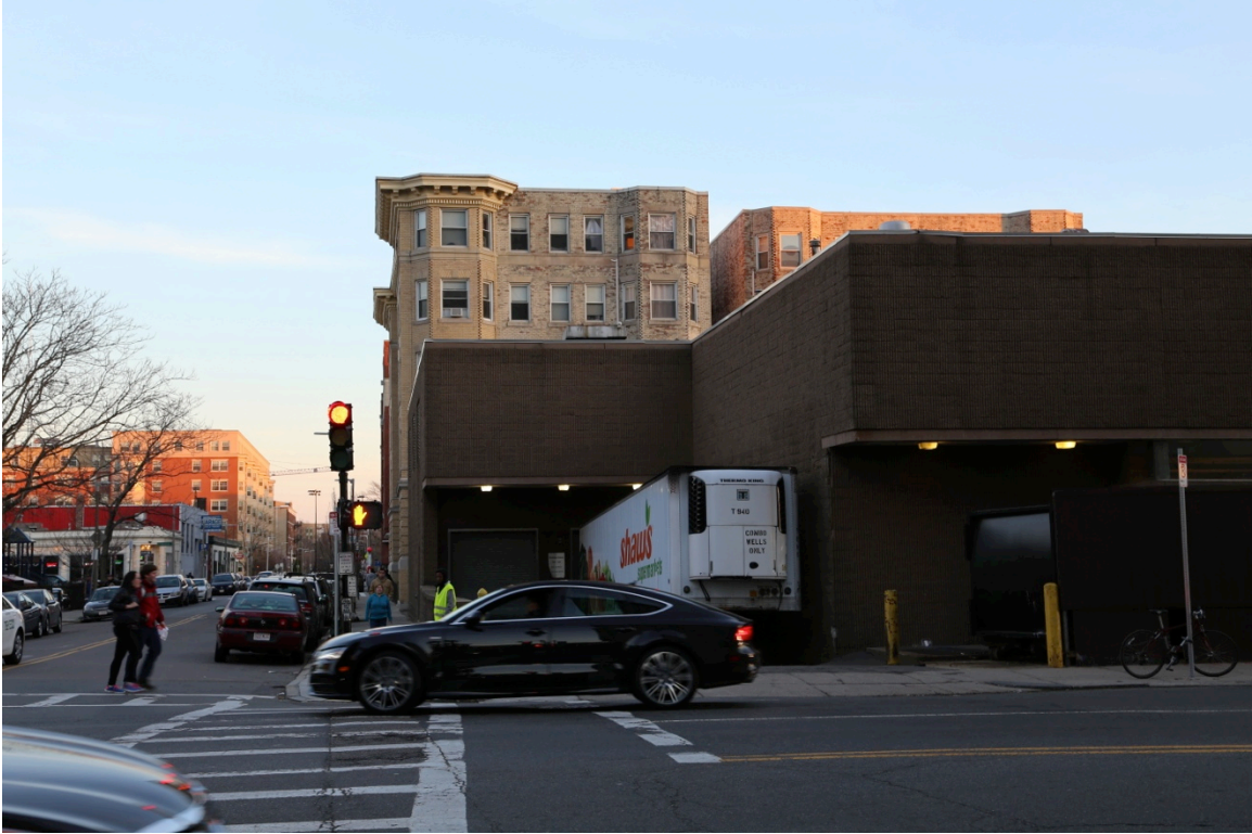
Figure 11. The building in Figure 9 visible from Boylston Avenue, including the visibly missing crown molding. Personal photograph.
