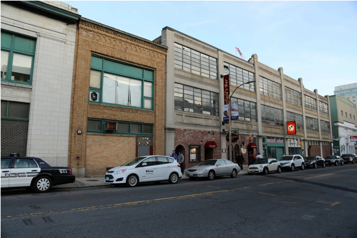
Figure 1. Dilapidated store fronts on Brookline Avenue. Personal photograph.
