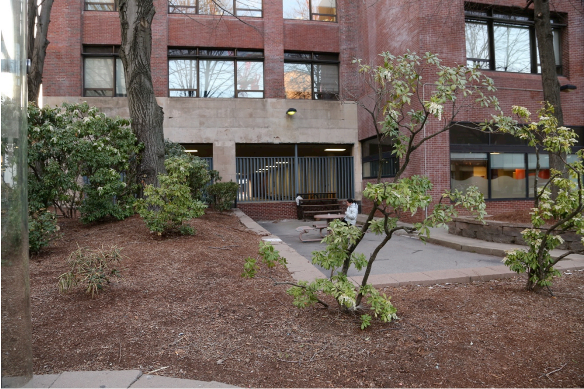
Figure 8. Parking garage attached to building with an entrance bricked closed and a repurposed driveway. Personal photograph.
