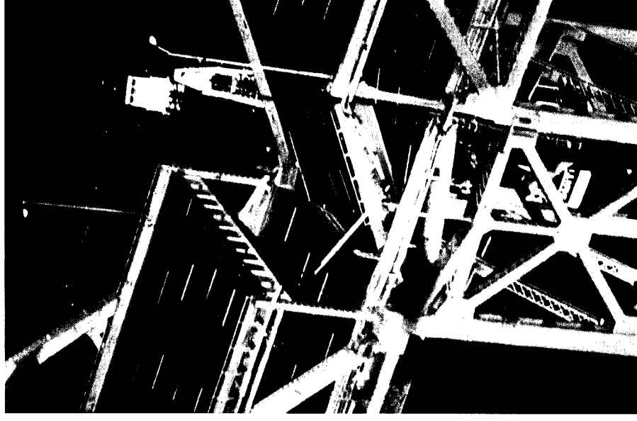
Figure 14. San Francisco-Oakland Bay Bridge: Failure of top slab in the 1989 earthquake.
