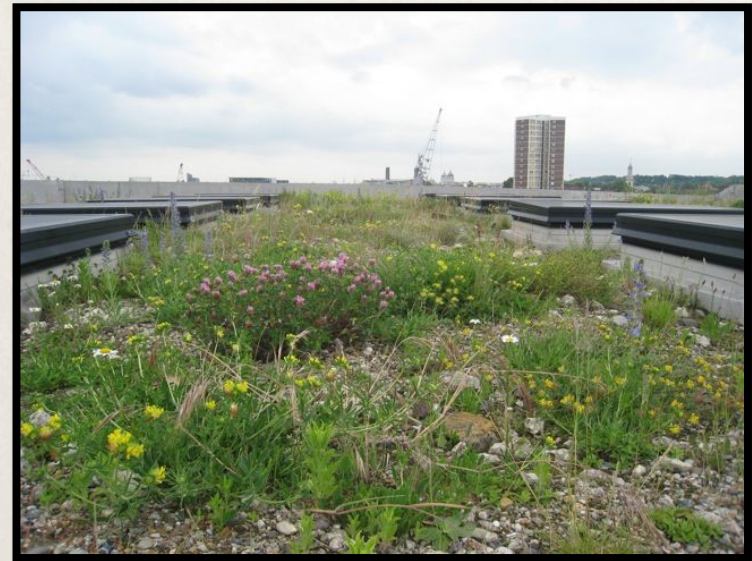
One of the first "brown roofs," constructed on the Laban Dance Center in southesastern London.
