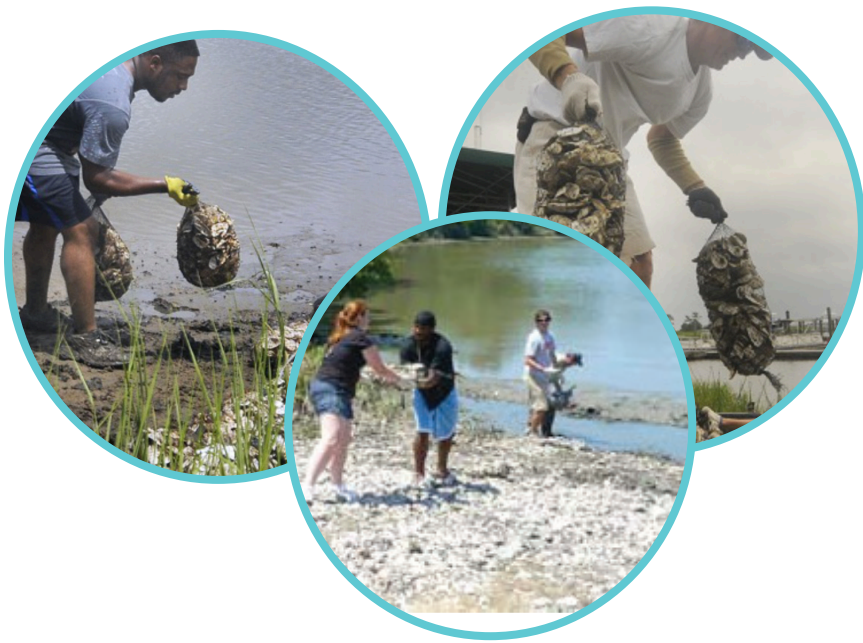
Figure 3: Volunteers build oyster reefs using mesh bags filled with oyster shells: Image Neil B. Chambers
