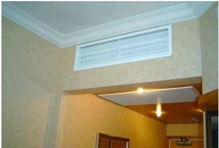
Figure 7-9 Example of installed Halton chilled beam
