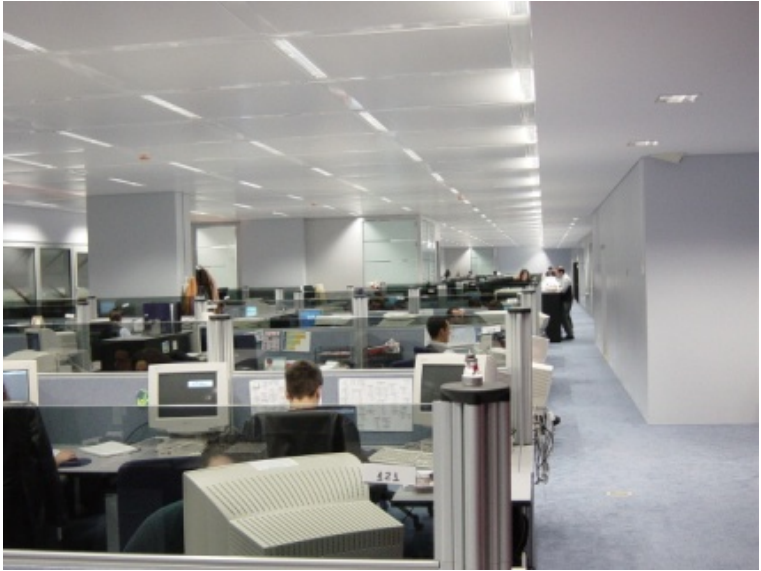
Figure 7-3 Example of installed radiant ceiling
