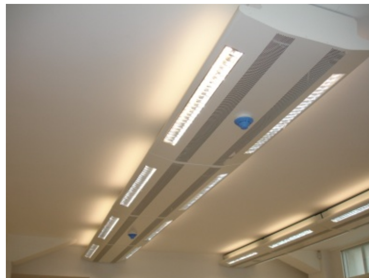
Figure 7-6 Example of installed chilled beam
