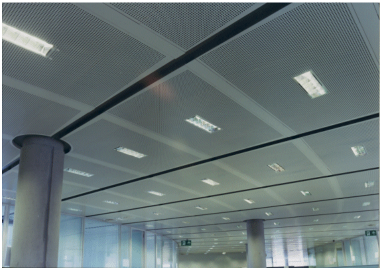
Figure 7-2 Example of installed radiant ceiling
