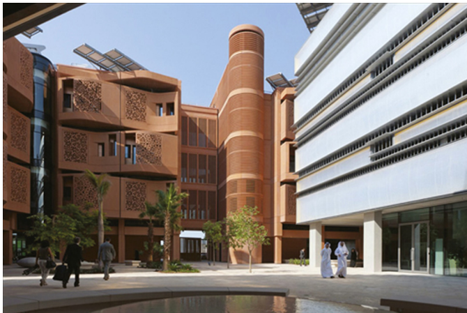
Fig. 5. Masdar Institute residential buildings (left) and laboratories (right).
