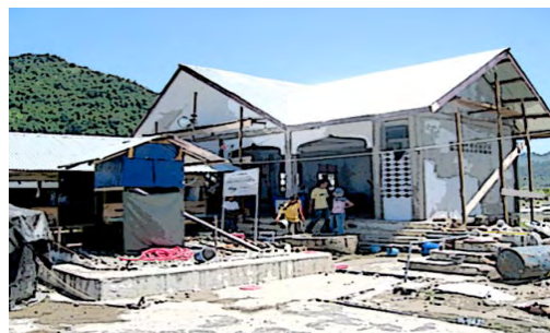
Mosque being repaired was workshop location.
