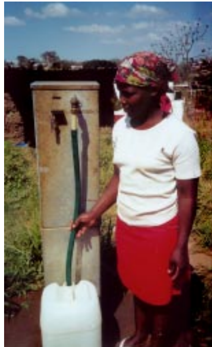
An automated standpost in which a user inserts a pre-paid card.
