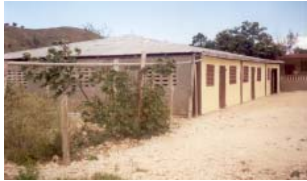
Figure 6.9: Roof Draining to Cistern
