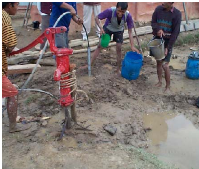
Figure 5-1. Construction of a Tubewell
