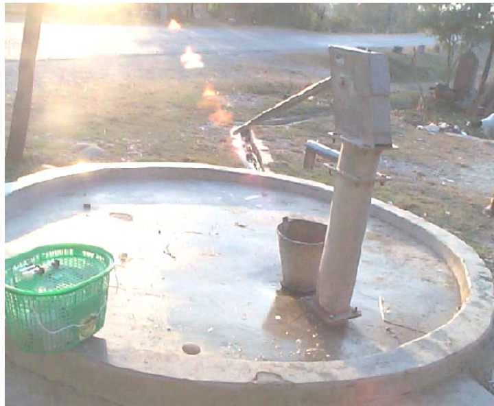
Figure 2-5. A Lift Tubewell
