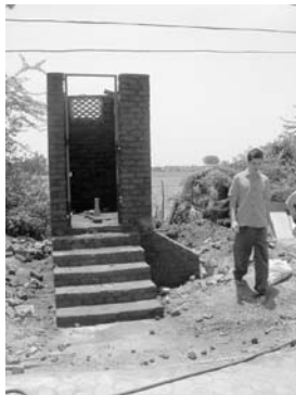
The demonstration Ecosan unit near completion.
